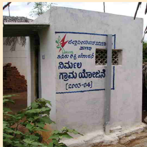
◀ A toilet constructed under NGY, Kabbigere (Koratagere)
