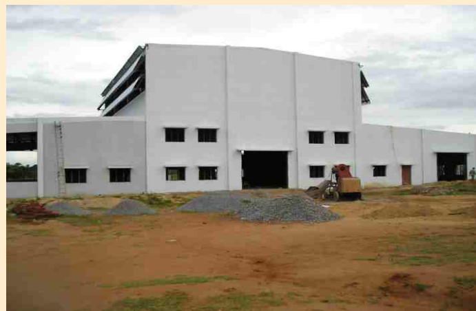
Gasifier building under construction, Kabbigere (Koratagere).
